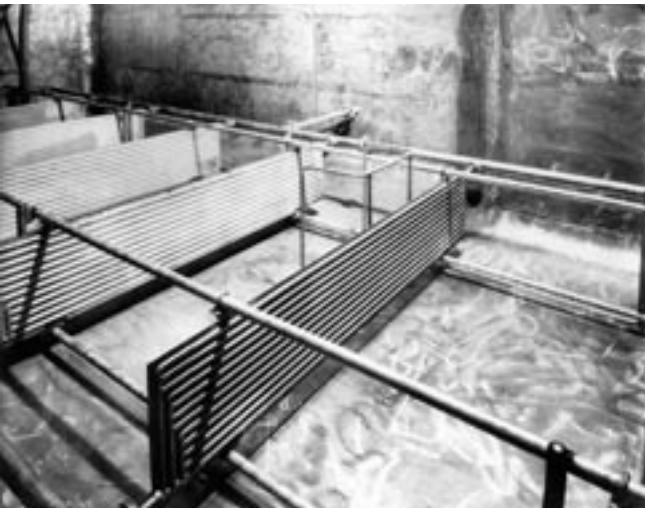
Fig. 65-3 The stainless steel PLATECOIL shown here are in a large compartment of a food products tanker. They are used for heating or for cooling depending on the product being transported.
